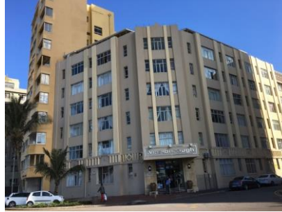
Some art deco decoration above the ground floor. Otherwise quite plain.
