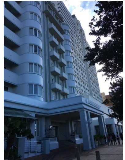
Art Deco streamline style (style moderne). Well maintained. Asymmetric entrance framed by rising bay windows on North end.
